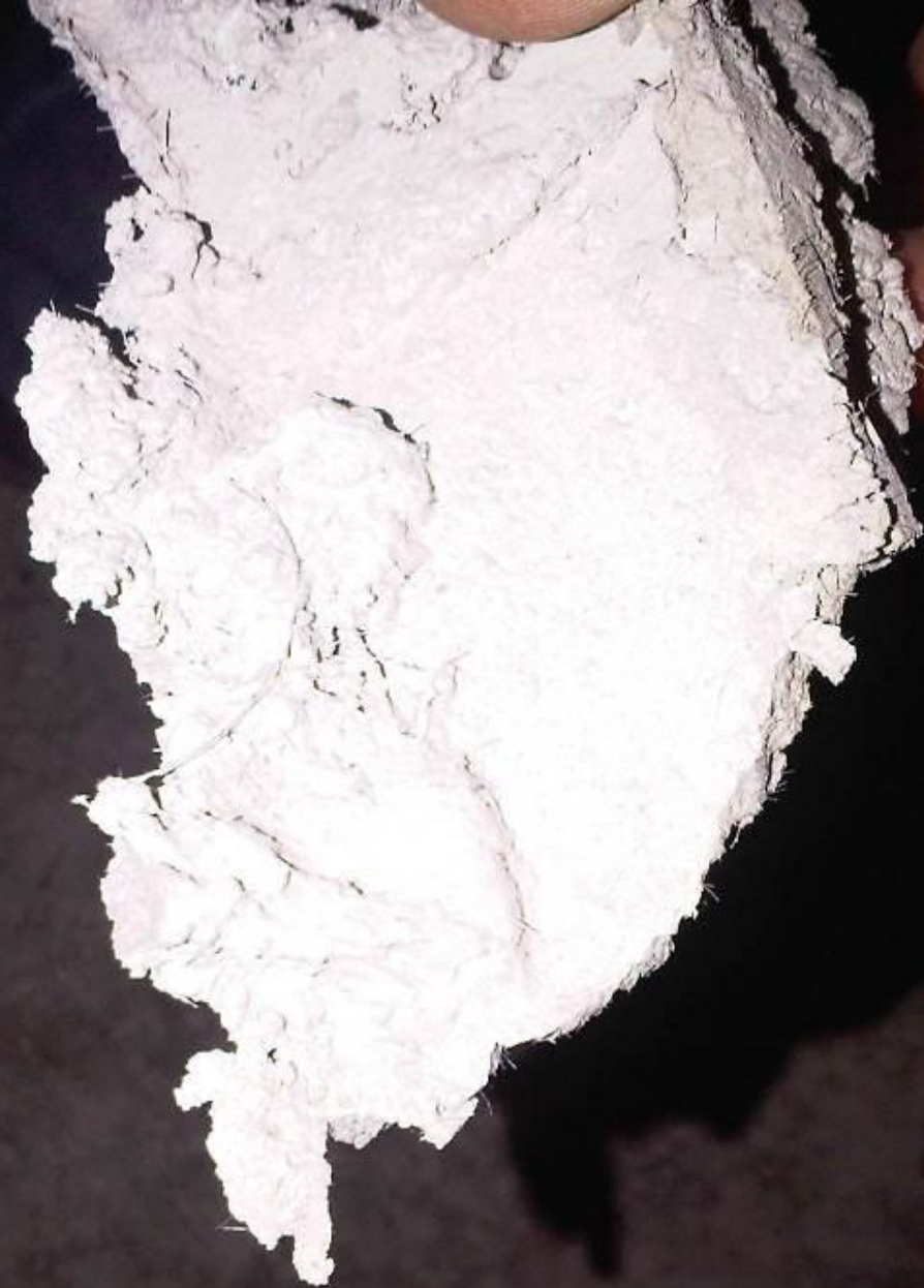
Asbestos cement/Hard coating on eg. Pipes(3)
